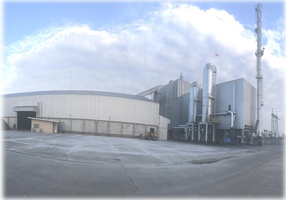
GPE (Industrial Waste Energy Power Plant) Installed capacity : 9.9 MW COD : 14 Jun 2018
